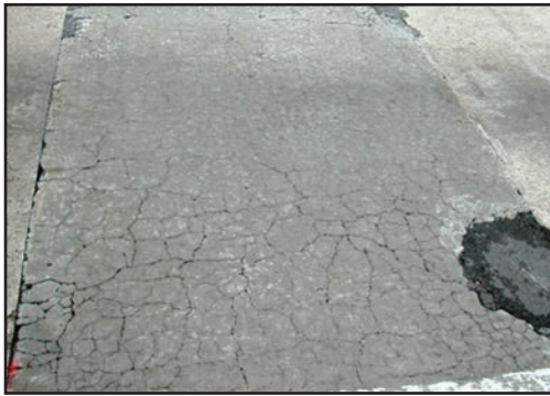
Cracking in Full-Depth Repair
